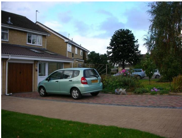
Fig. 12: High density housing with off-road car parking for more than one vehicle (Orchard Road)
